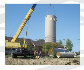
Completely water tight housing dimensions depend on the equipment to be installed into the sewage pumping station and on the required retention volume.
